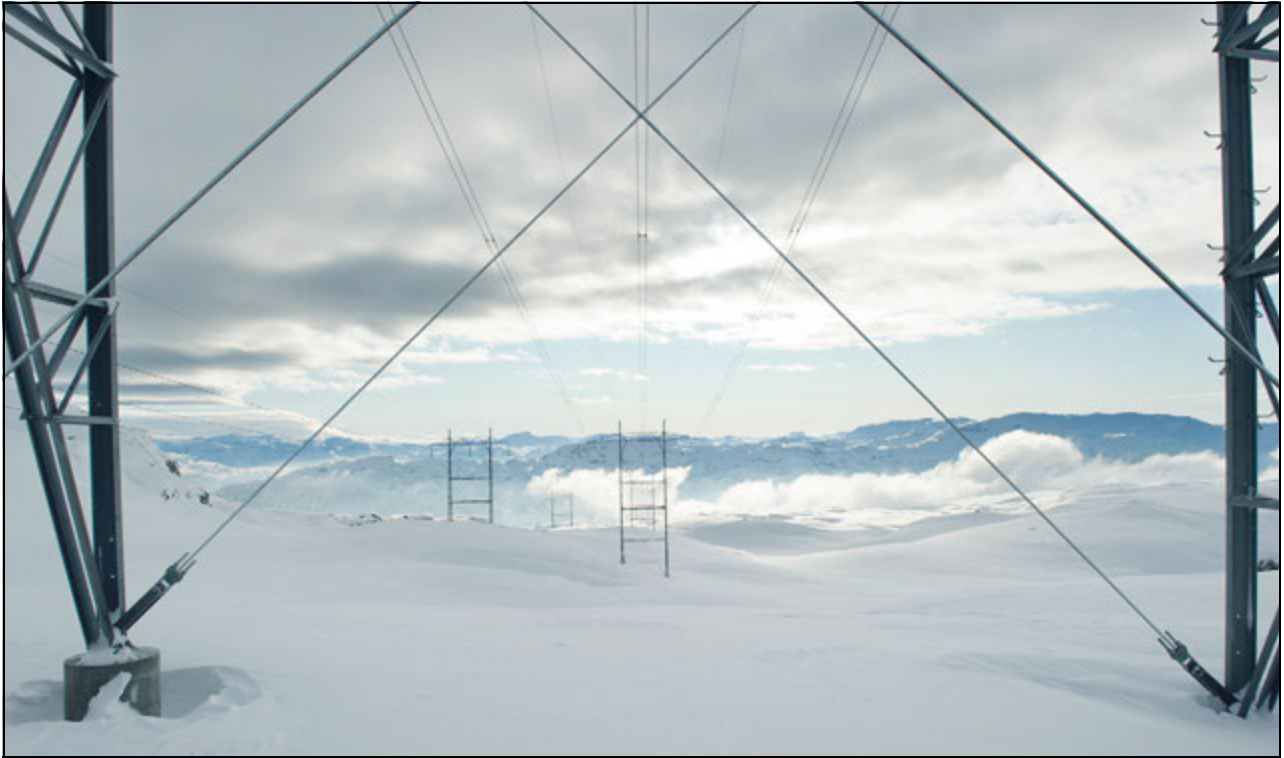
Figure 8.1 Power lines near the Hylsfjord
